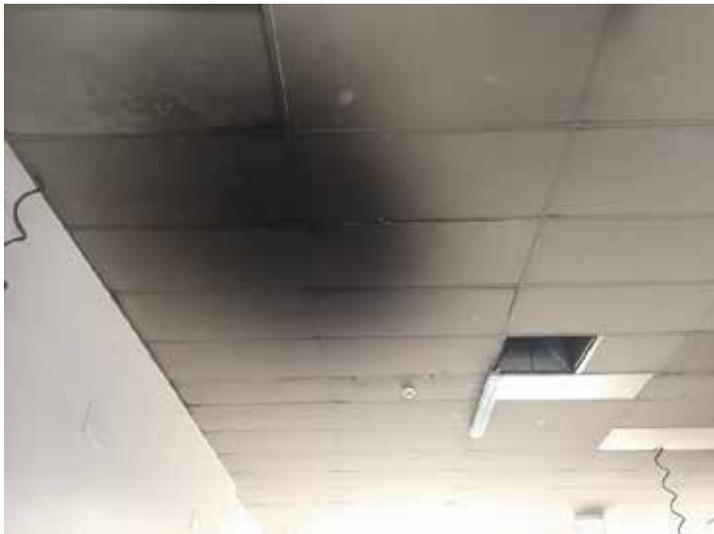
Figure 1. Diesel Particulate contamination of ceiling at St. Mary's Station December 2019
