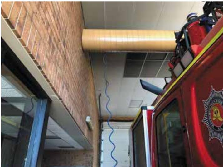
Figure 3. Figures 2, 3 and 4 identify that the Appliance Exhaust configuration and Local Exhaust Ventilation (LEV) system are substantially mismatched. Diametrically opposite configurations allow for diesel exhaust contamination of work environment and surfaces.
