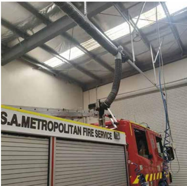
Figure 5. Mt Barker Station January 2020. The Point of Capture LEV system may provide for reduction in DPM but the efficacy of the system requires assessing to ensure appropriate design, flexibility in Appliance exhaust configuration and adequacy.
